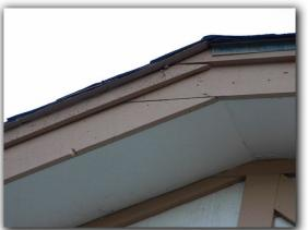
☑ Areas of the roof covering drip edge flashing were damaged or improperly installed and may allow water intrusion or water damage.
