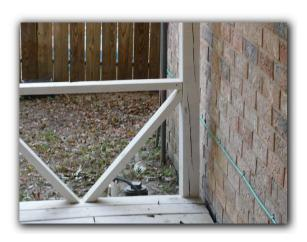
$\ \square$  Deck and patio cover ledge board should not be supported by brick or stone masonry according to current building standards.
