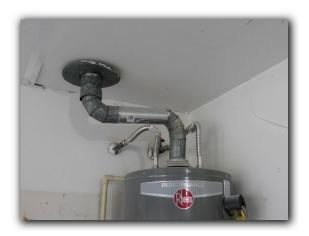
☑ The water heating equipment TPR drain line was not plumbed to the exterior.
