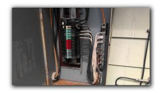
$\square$  The electric service panel cabinet cover plate or dead-front screws were observed to be missing and should be replaced with the proper screws as needed.
